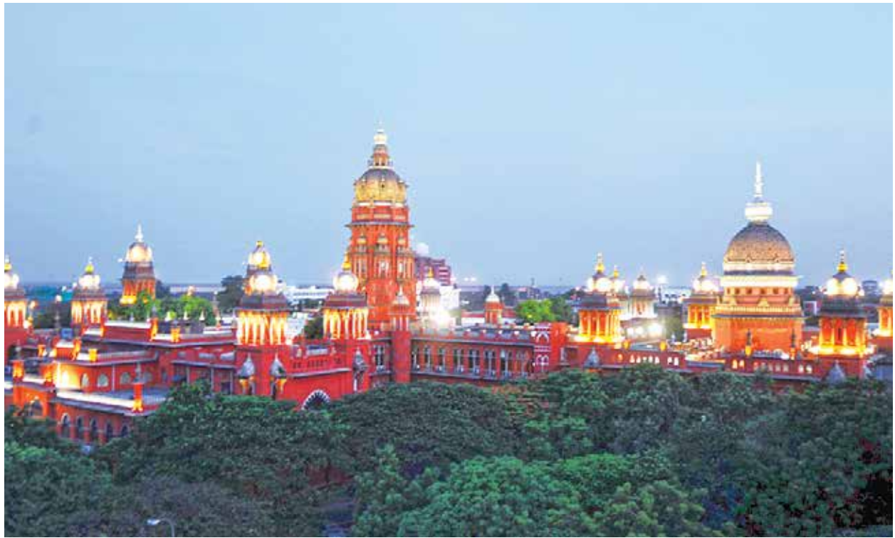
Illuminated view of Principal Seat of the High Court
