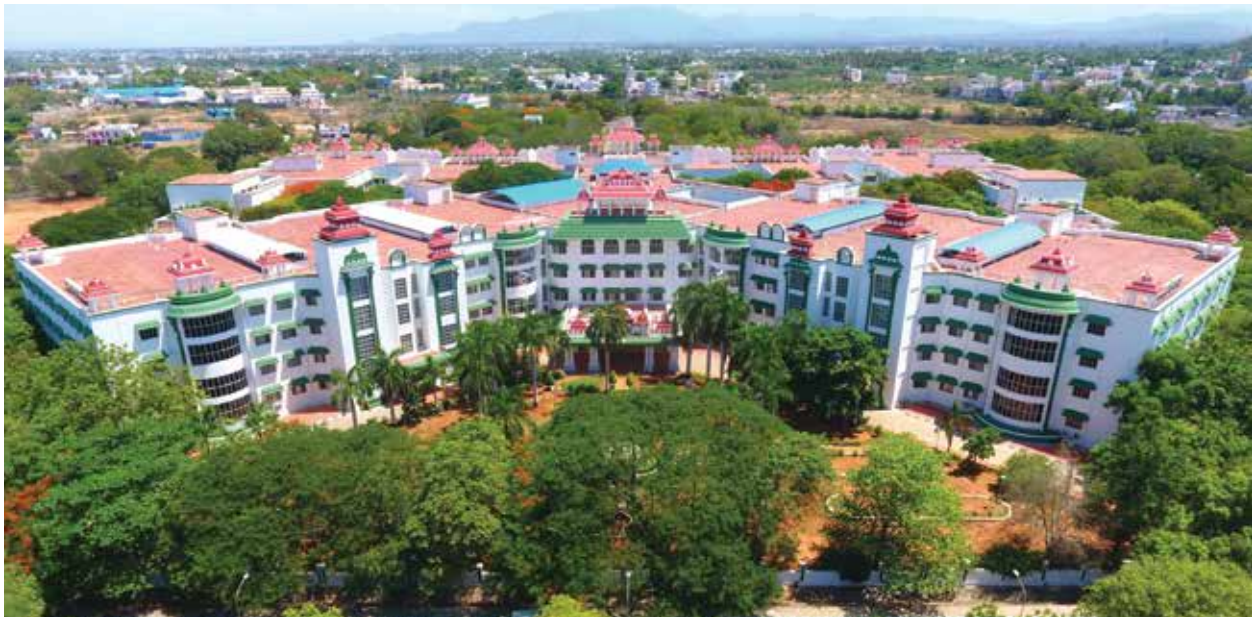
Aerial view of Madurai Bench of the High Court
